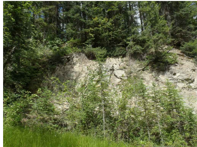
LOOKING TOWARDS WOODS ABUTMENT
