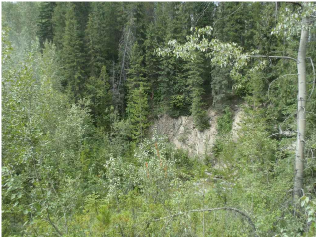
LOOKING AT WOODS ABUTMENT FROM TOWN ABUTMENT
