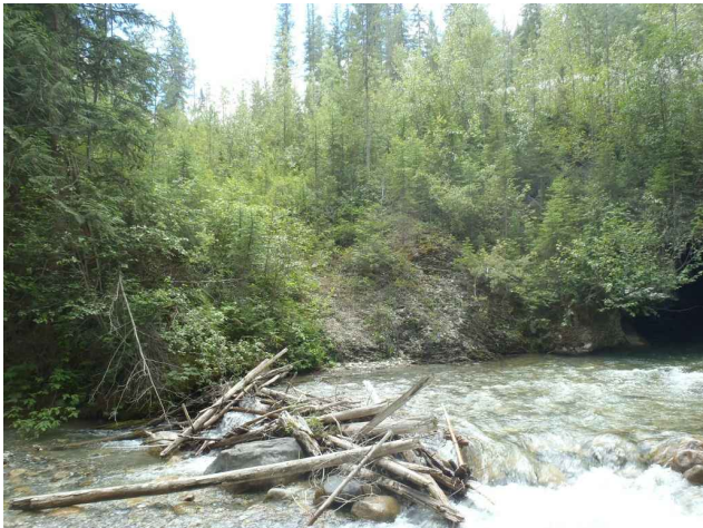
TOWN ABUTMENT ON SLOPE LEFT OF PHOTO
