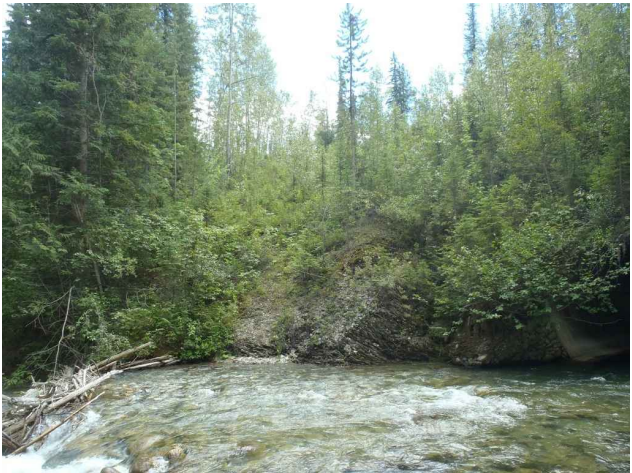
LOOKING TOWARDS TOWN ABUTMENT
